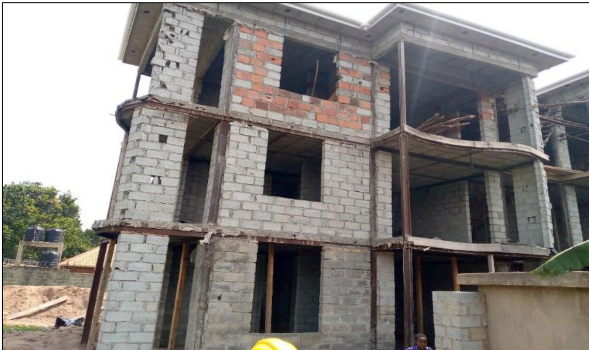
Figure 30: Structure constructed using the STC Composite in Kavumba village, Wakiso
