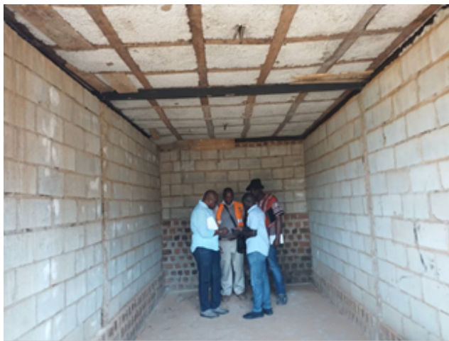
Figure 2-8: Masonry infill walls
