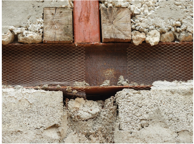
Figure 2-19: No contact between beam and its supposed lower column section
