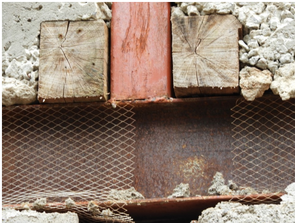
Figure 2-13: Column loading a beam
