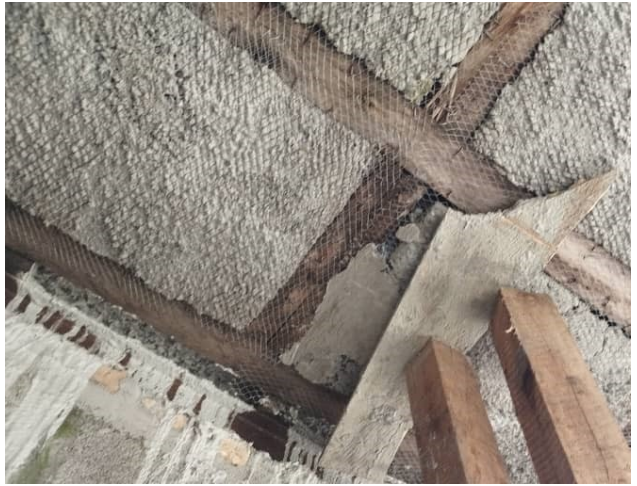
Figure 2-7: Failed Ceiling panel
