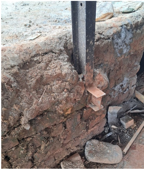
Figure 2-21: Superstructure to substructure connection
