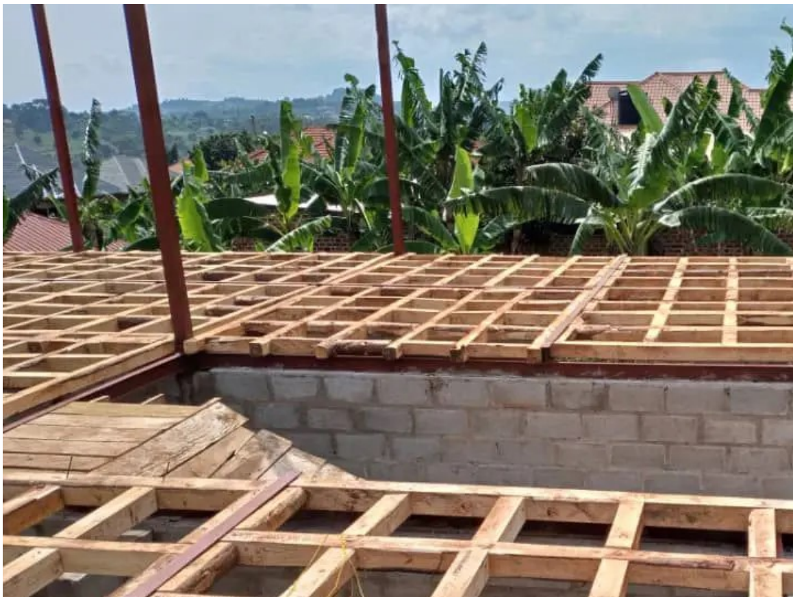
Figure 1-2: Timber framework in typical STC Slab construction (Credit: Enock Kirabo)
