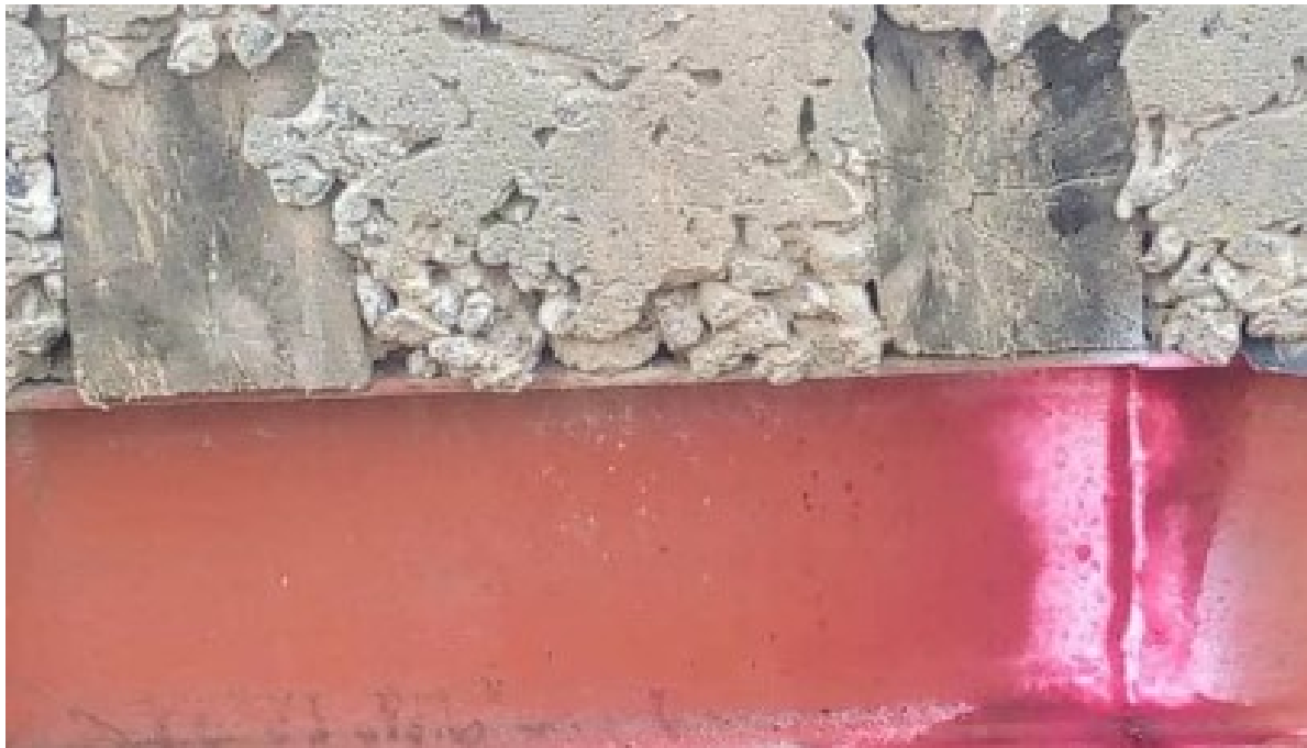
Figure 7-19: One of the few acceptable butt welds
