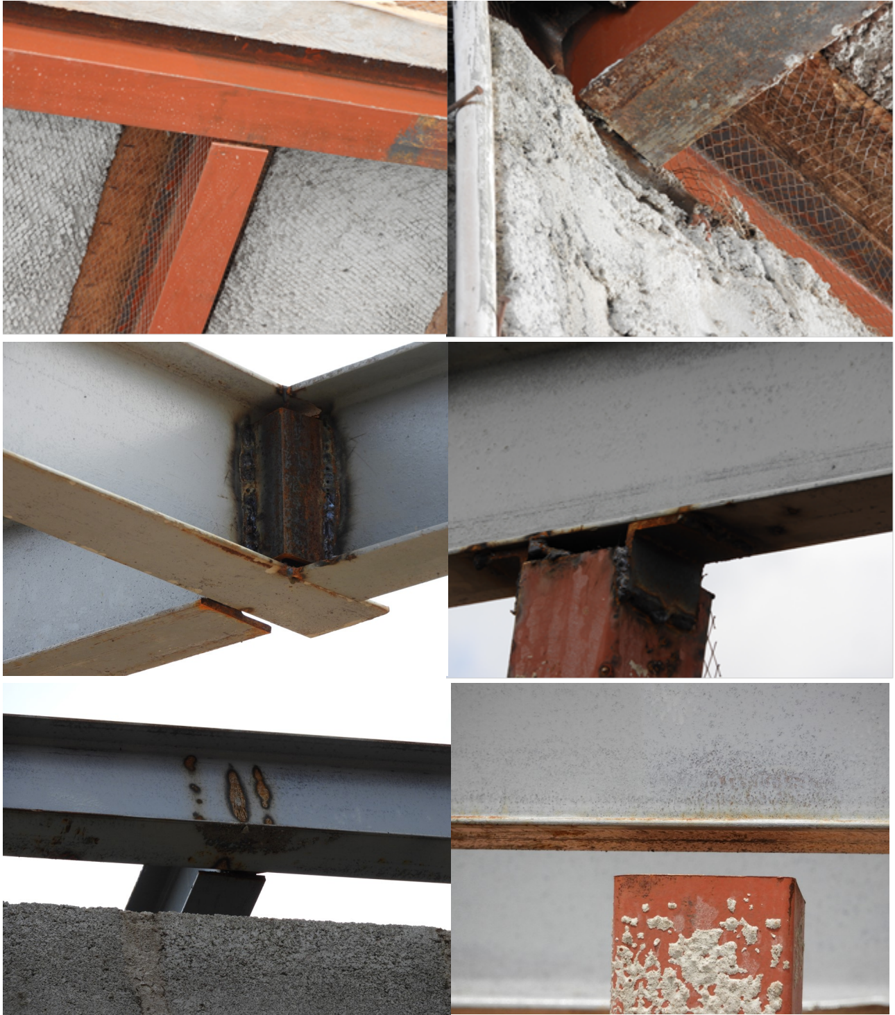
Figure 2-18: Gaps left at 'connection' points
