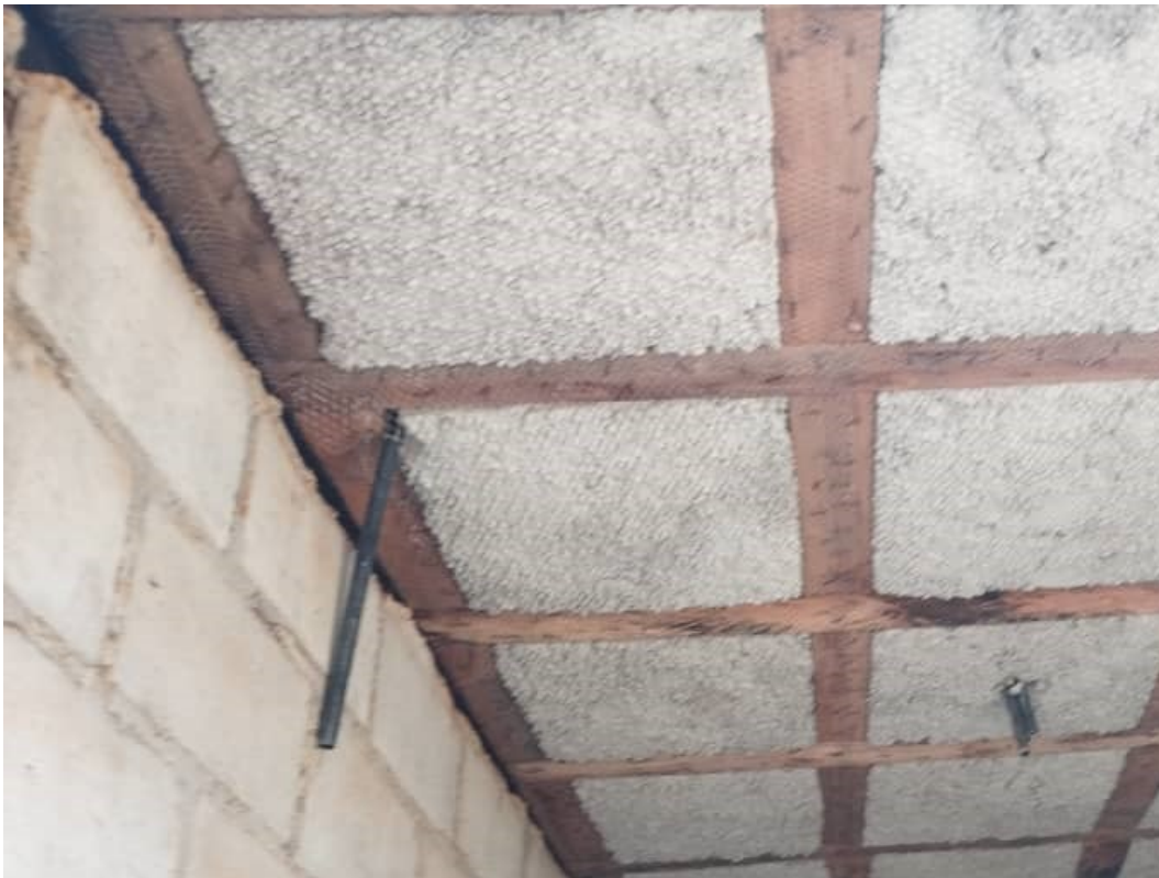
Figure 1-6: STC Slab after construction
