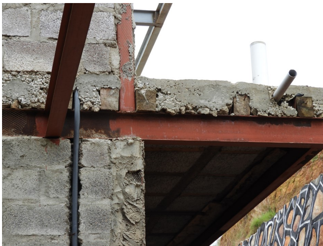
Figure 2-14: Offset beam from column position, loading another beam
