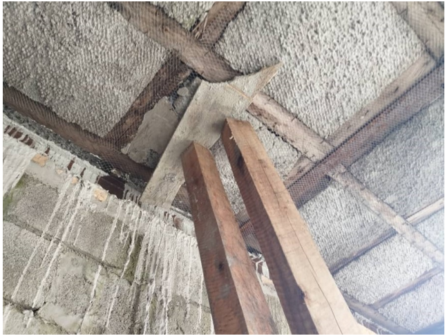
Figure 2-7: Failed Ceiling panel
