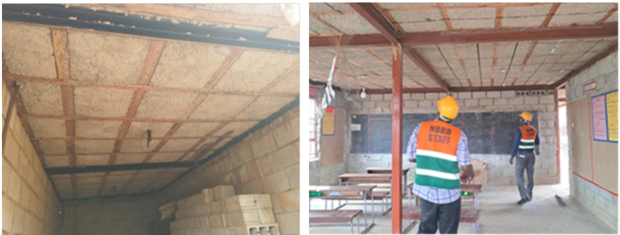
Figure 2-5: Soffits of STC slab
