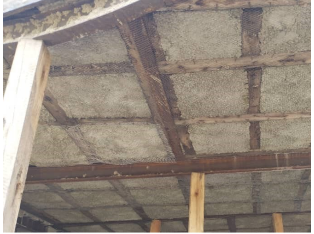
Figure 2-6: Propping of steel beams with timber during construction
