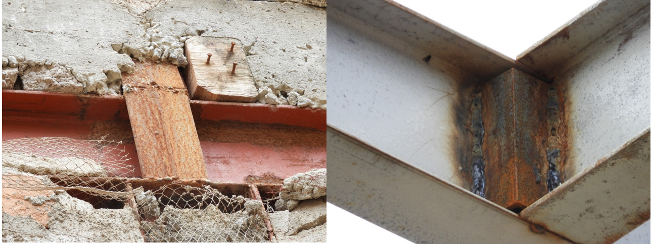
Figure 2-15: Unconventional connections
