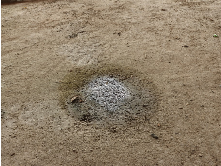
Figure 2-12: Construction stage leakage through slab and dampness at bottom of slab
