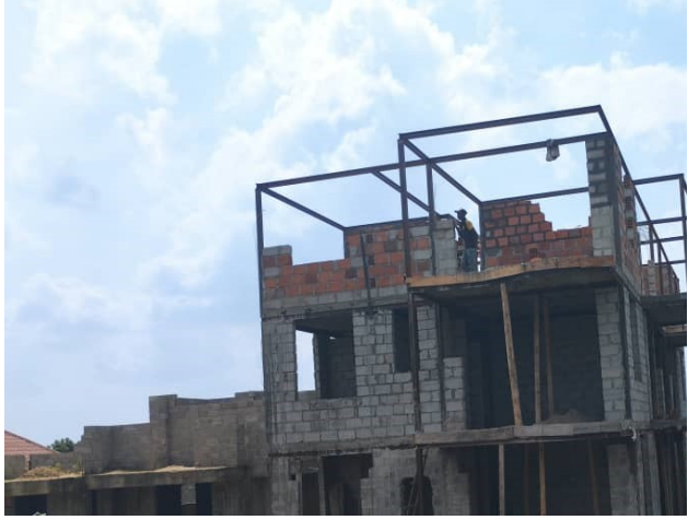
Figure 2-6: Propping of steel beams with timber during construction
