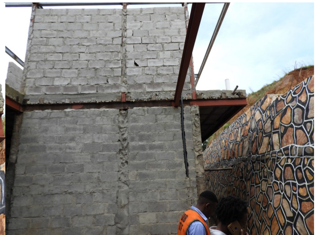
Figure 2-14: Offset beam from column position, loading another beam
