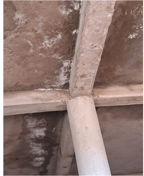
Figure 2-12: Construction stage leakage through slab and dampness at bottom of slab
