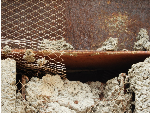
Figure 2-19: No contact between beam and its supposed lower column section
