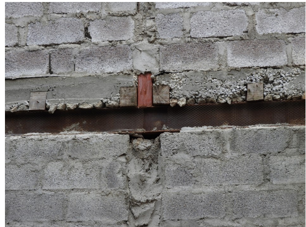
Figure 2-13: Column loading a beam
