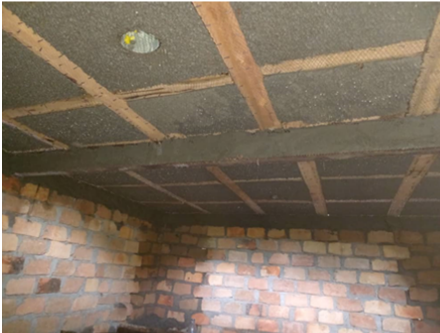
Figure 3-14: Underside of the STC Floor system investigated for fire resistance
