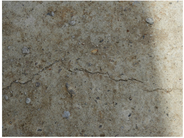
Figure 2-20: Cracking in the Concrete Slab
