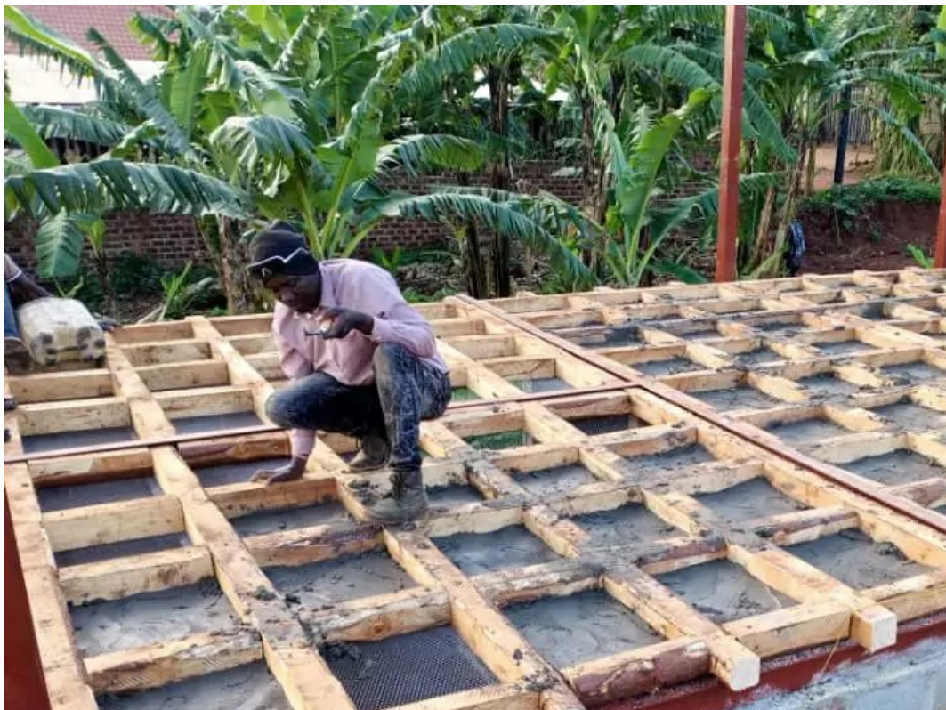
Figure 1-4: Pricking up mortar is applied from the top (Credit: Enock Kirabo)
