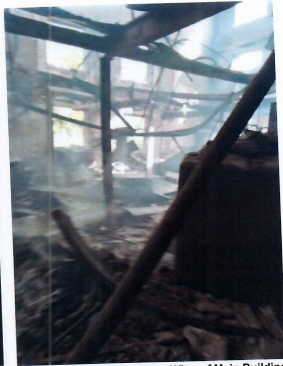
Figure 9: Smoke in Northern Wing of Main Building
