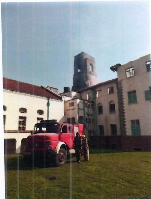
Figure 6: Smoke Coming Out of Tower of Main Building
